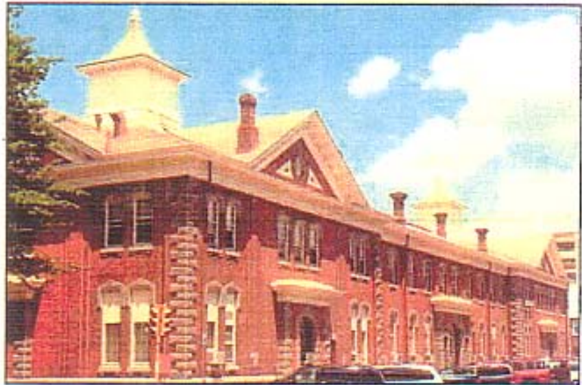
This before photo shows historic Building 1 that houses Public Works Department Pennsylvania. The building has a grand, high style and is a detailed example of Italianate architecture, but it was much in need of repair.
