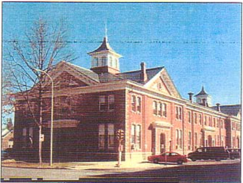
This after photo shows repairs completed to the roof with beauty intact.
